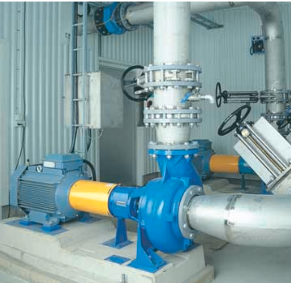
These FB pumps at Stora Enso, Sweden, are pumping the leftovers from paper making. The liquid contains fibre sludge.
