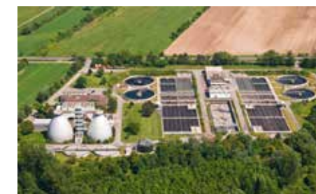
Waste water and sludge treatment / municipal waste water
